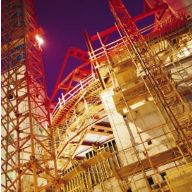
TAIB Tower (scheduled for completion in December 2002) Manama, Bahrain
